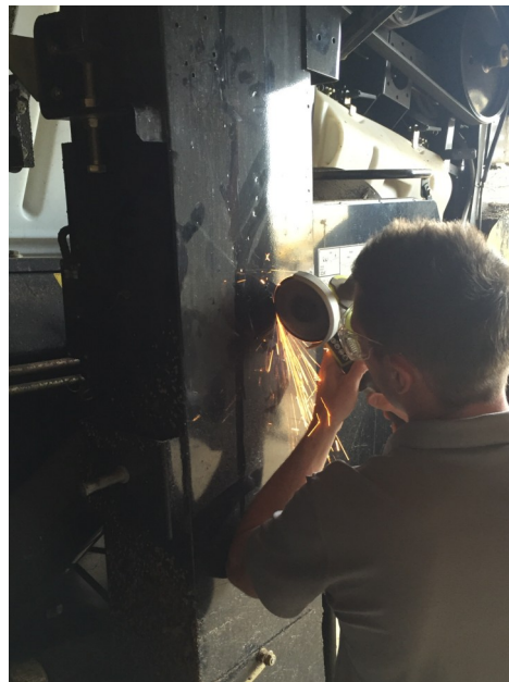
Fig. 2.2. Clean Grain Elevator. Top Inlet Cutout and Holes
