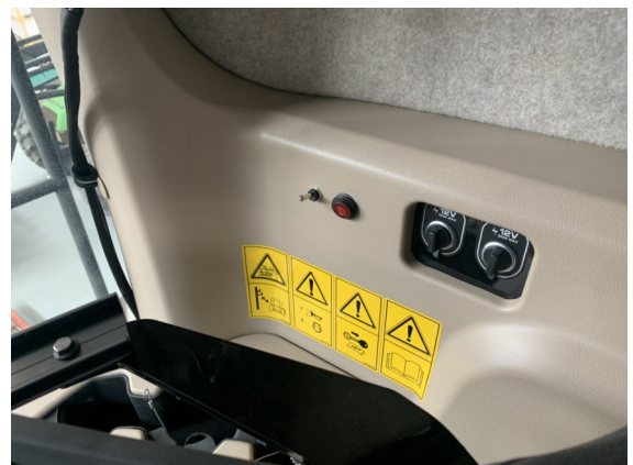
Fig. 2.18. ON/OFF Switch installation.
